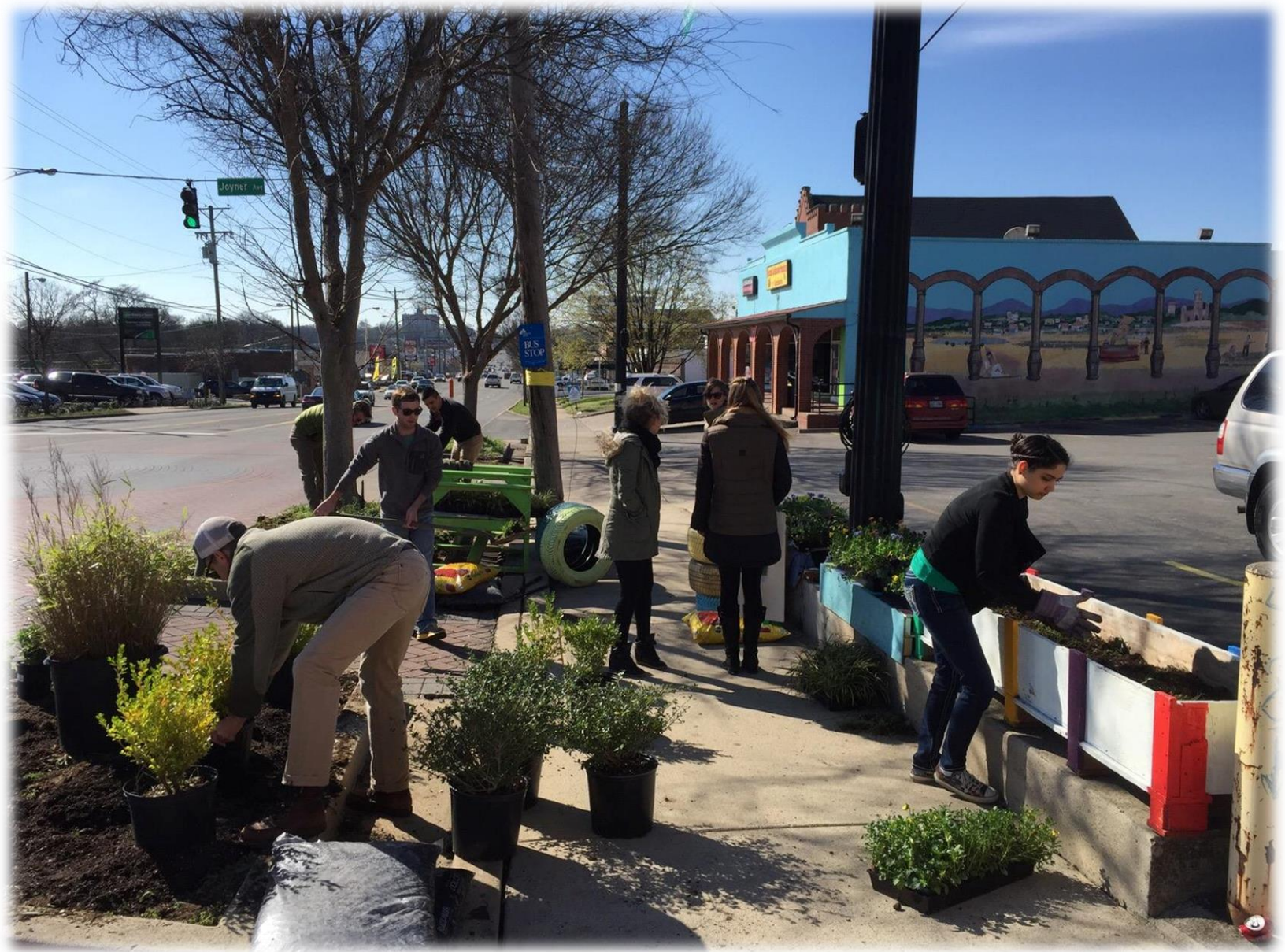
Turbo: Bus Bench Installation next to La Hacienda
